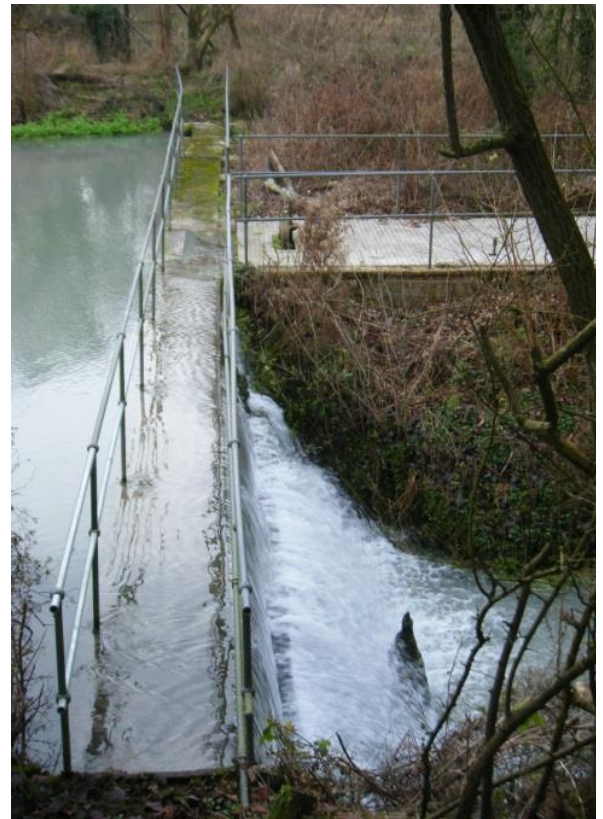
Fig 3. The dam and its location. The brook is in flood ( \sim 0.8\text{m}^3/\text{s} ) and is overtopping the dam, the dark spike down-stream is the top of the drawdown valve. The power house is the vegetation covered protruding structure.
